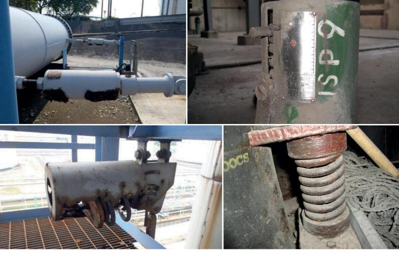
Corrosion is the real destroyer of pipe supports, as the photos show. With many units operating in very harsh conditions, it is particularly important to regularly review their condition across the site to identify and isolate problem supports, or pipework corrosion and damage, before it becomes critical.
